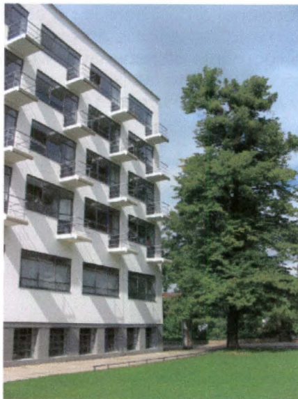
Figure 16: Dormitory Cantilevered Balconies
