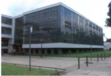
Figure 15: View from Street
