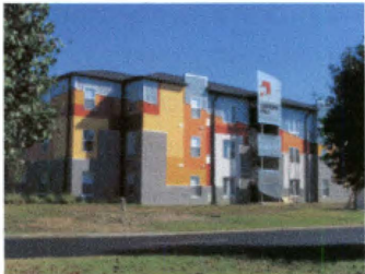
Figure 22: Existing Student Housing
